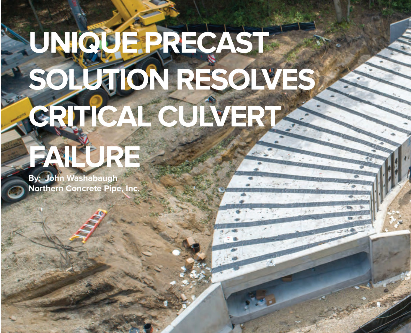
Aerial photo of completed installation of unique precast box culvert
