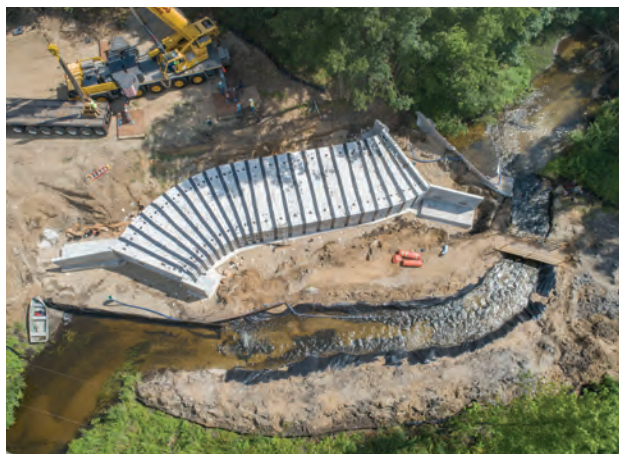
Yet another overview complete with stream diversion, and contractor foot bridge
